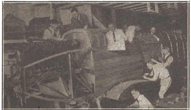
"Mass" production in 1921. Of all-wood construction, this Douglas DT was used by Naval Air Service for torpedo duties. Power plant was a 400-h.p. Liberty on spruce engine mounts.
